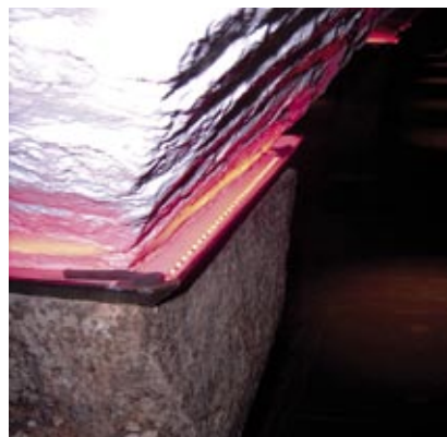
Figs. 6 and 7. The LINEARlight Colormix LED modules are discreetly positioned on the pillars
